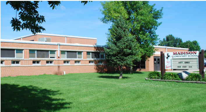
Madison Elementary School in Fargo, North Dakota adopted Hydromx heat transfer fluid for their 75-ton capacity chiller.
